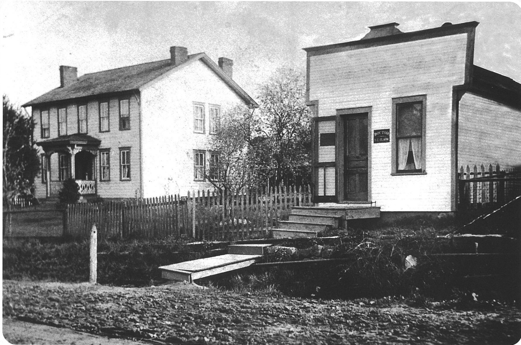
The office of Worthington native son Dr. Omar C. Clark was located immediately adjacent to his childhood home at Main and Bear Streets. The sign beside the front door reads, "Dr. O.C. Clark." Notice the marked contrast between his parents' spacious frame residence (left), and Clark's tiny medical facility with its lone window. The uneven terrain, lop-sided steps, precarious wooden walkway and rudimentary hitching post bear witness to the state of development common in rural areas in 1906. From the collection of Lois E. Reed.
